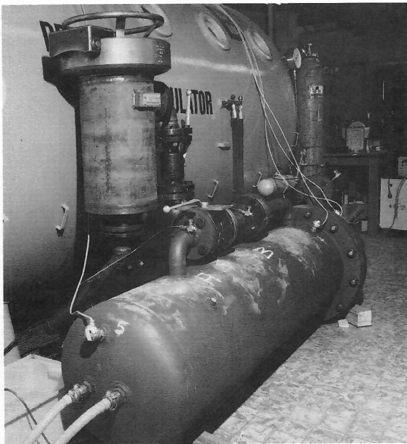
Fig. 10.17. Cylindrical carbon dioxide filter unit by Dräger, installed vertically, with pressure-proof circular bayonet lock for replenishment.
