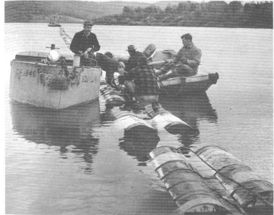
Fig. 14. Floatation method: barrels are used to float this intake water system. (Cast Iron Pipe Research Assoc.)
