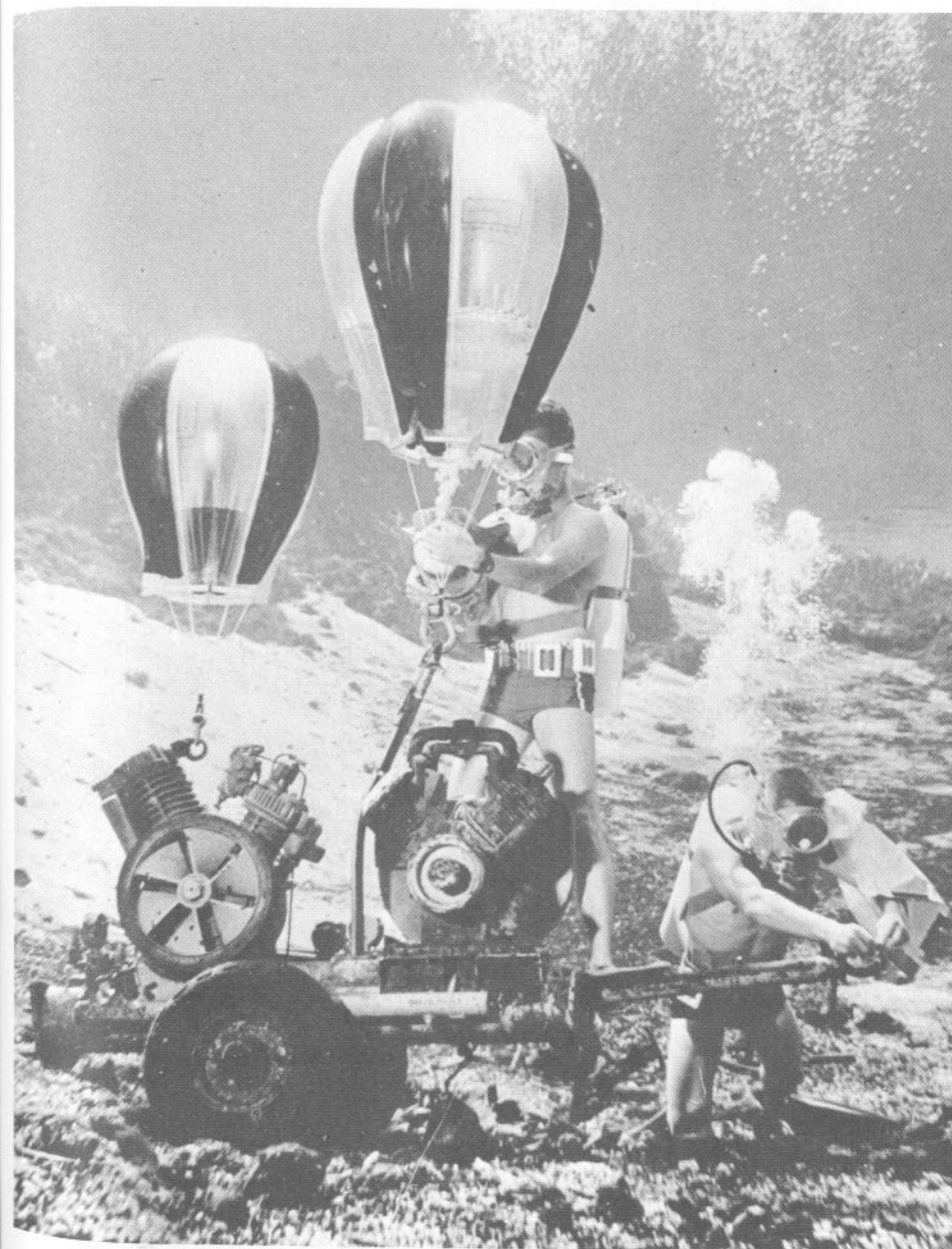
Fig. 7A. Lifting bags being used to raise a sunken compressor. (Hypro Diving Equipment Co.)
